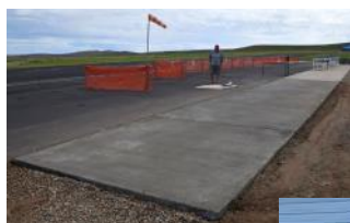
Left and below our newly poured concrete pads at the field.
