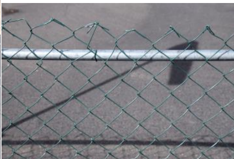
New fencing to replace old safety fence material. This will last longer and also be easier on aircraft that collide with it.
