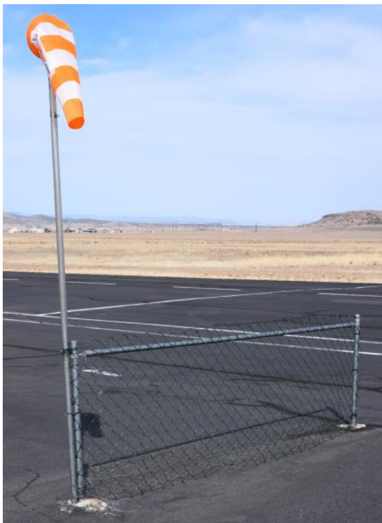
New fencing to replace old safety fence material. This will last longer and also be easier on aircraft that collide with it.
