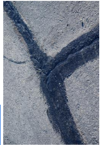
Runway cracks now sealed.
